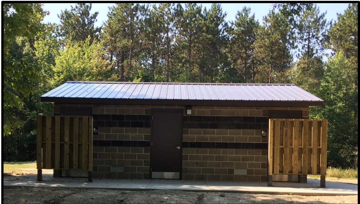
New Restroom with Showers at Sherwood County Park
