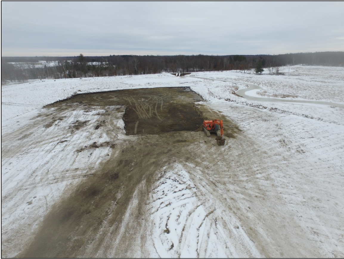
Sherwood Lake Dredging – January 2016
