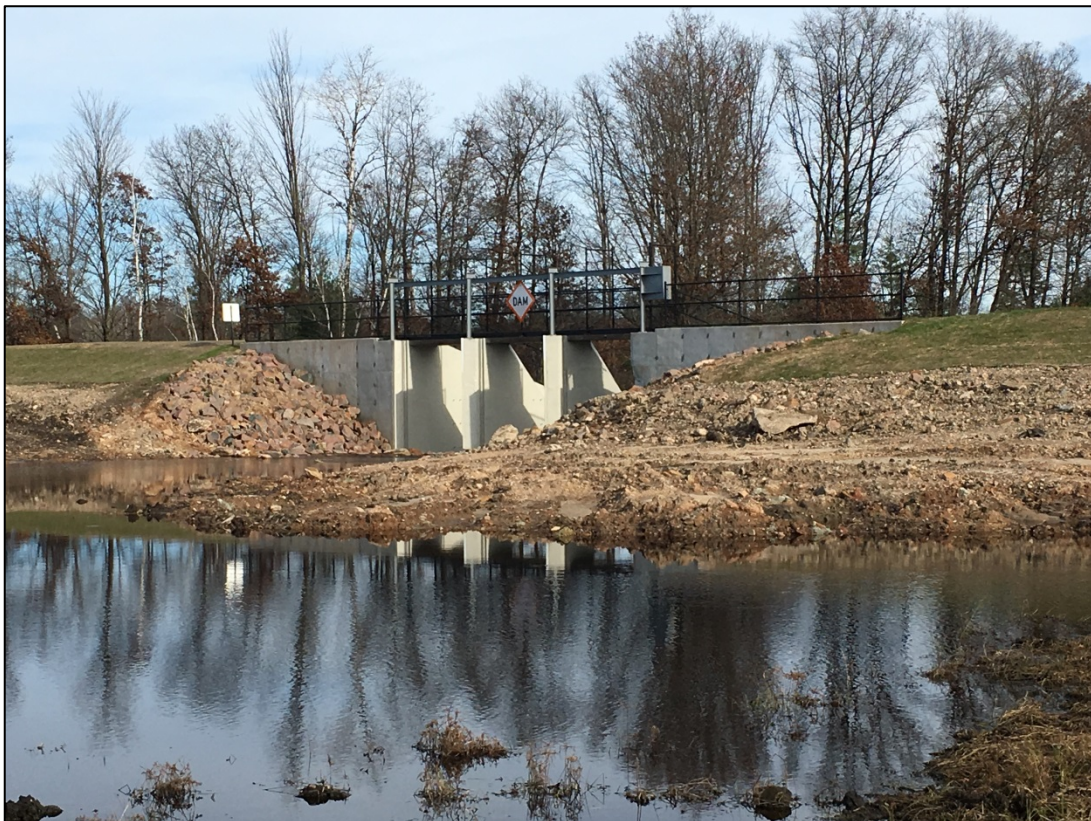
Sherwood Lake Dam
