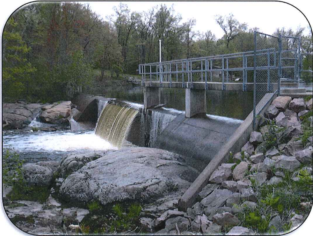
Snyder Lake Dam
